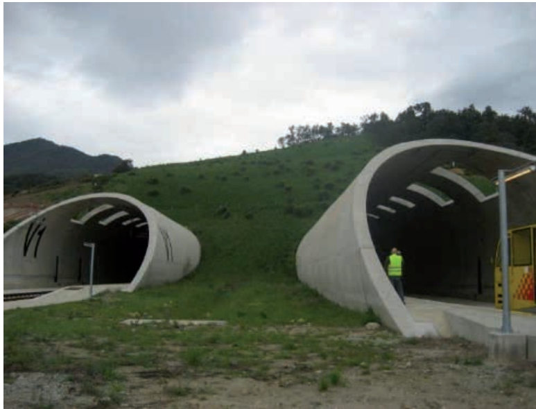
Figure 6. North Porous Portal. Perthus Tunnel.
