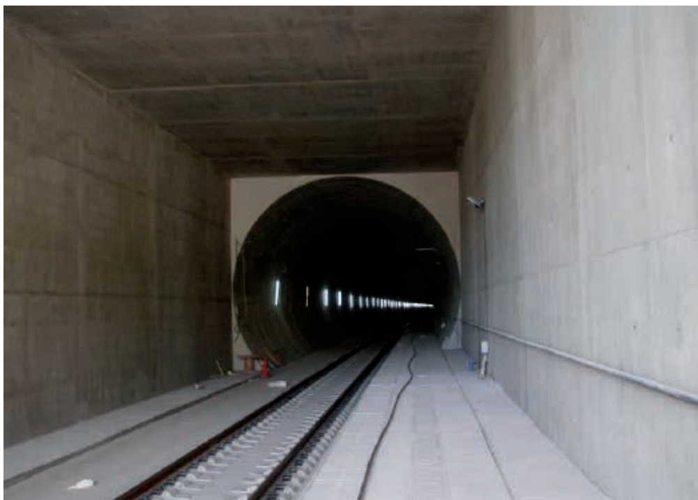
Figure 8. Inner of North Portal of La Cabrera Tunnel.
