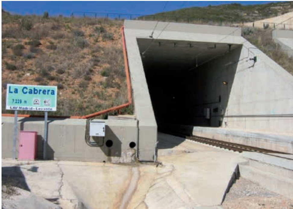
Figure 7. North Portal of La Cabrera Tunnel.
